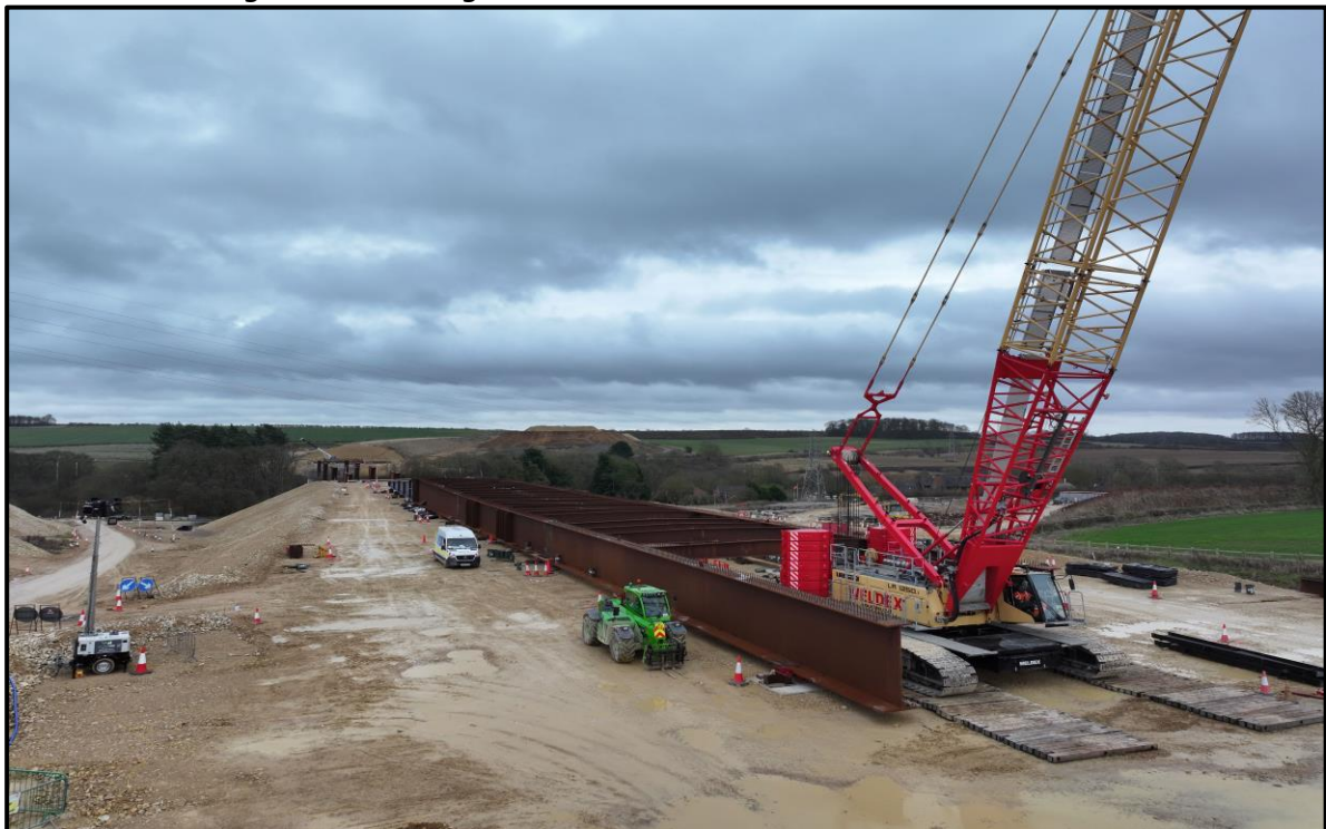
GSRR – First Bridge Section being Fabricated on Site
