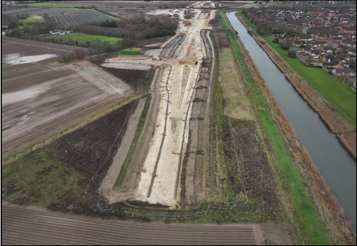
SWRR – Aerial View Looking East along Vernatt’s Drain
