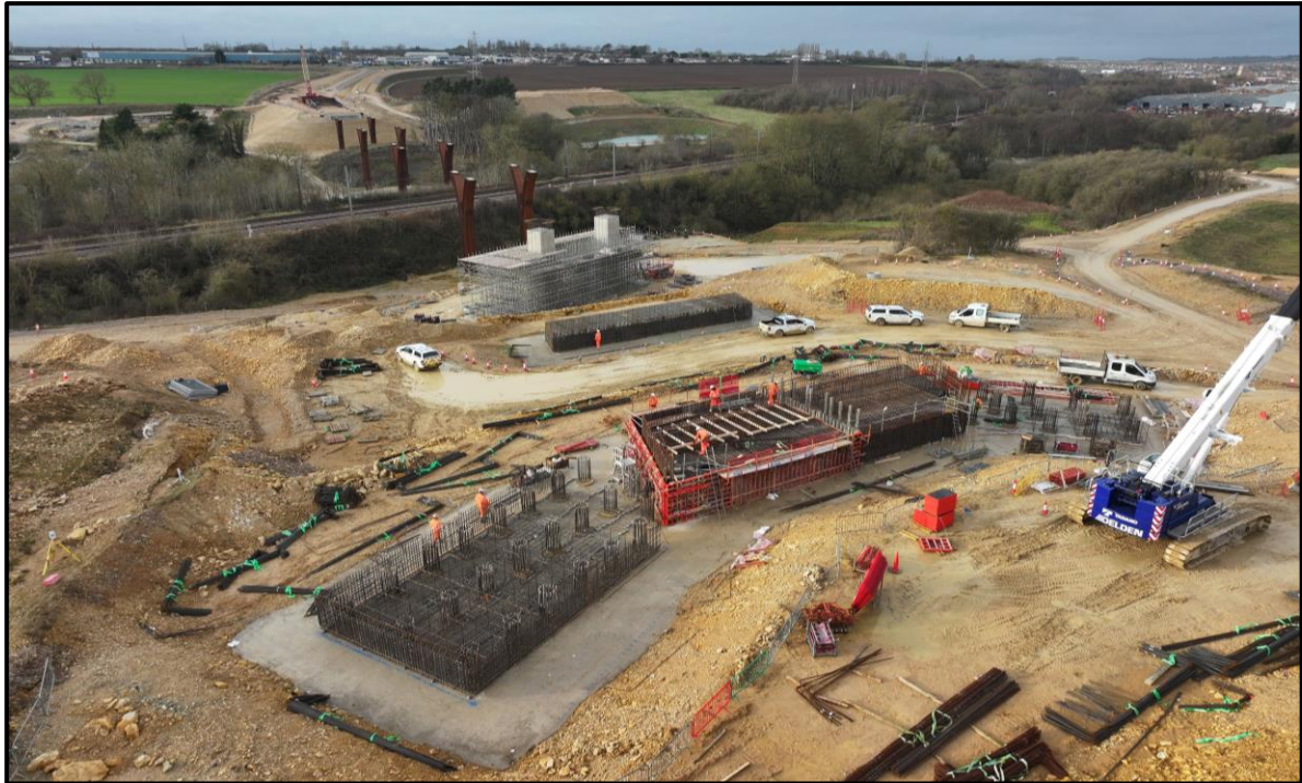
GSRR – Pier Progression of Extended Bridge Eastern Abutment
